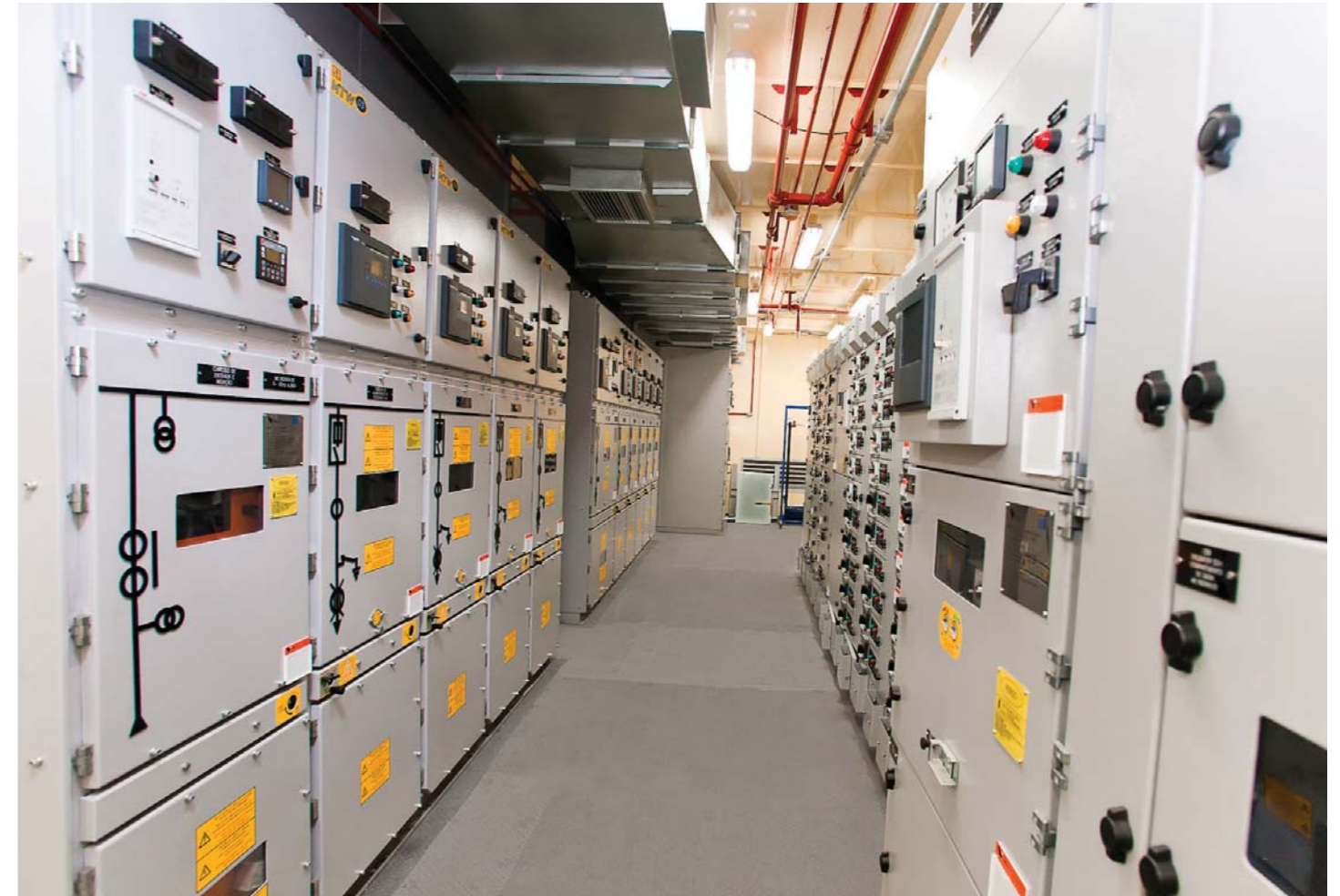
LV and MV Switchboards inside "E" House
