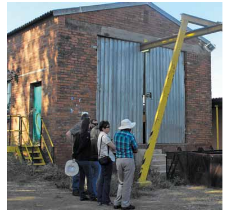
▲ Hot water treatment plant at Gledhow Mill
