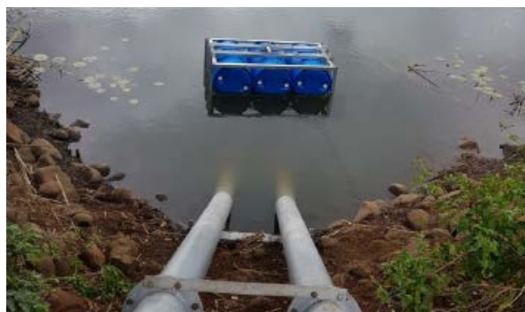
▲ Sediment dam with pump suction intake on a float
