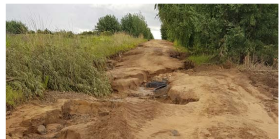
▲ Figure 3: Unusable road due to soil erosion.
