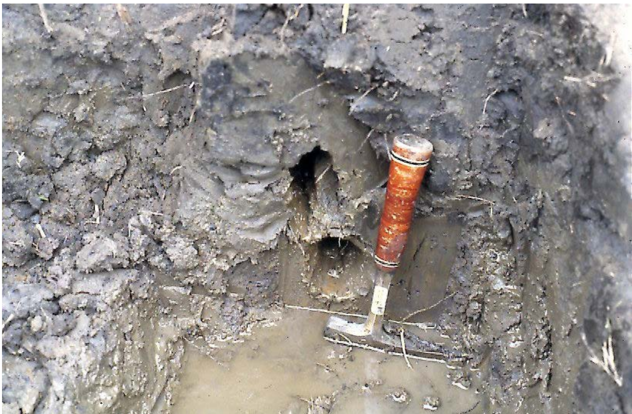
▲ Figure 1: A mole drain at a depth of 450 mm in the gley horizon of a Rensburg soil form.
