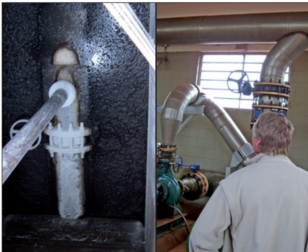
Figure 8.11. Accumulation of potassium chloride from vinasse on the pipework of a vinasse reservoir (left). Vinasse pump house with stainless steel piping to minimise the effects of corrosion on maintenance (right).
