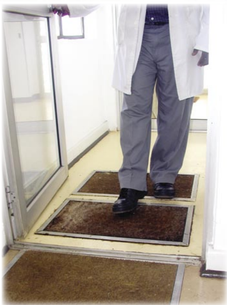
Three stage system of airlock doors and disinfectant footbath mats are in place to prevent the escape of pathogens.
